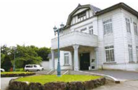
Misato Town Library, Gakuyukan
